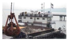
workboats. The contractor used two total stations on the shore in order to position a workboat in the proper location to dump the load of rocks. An additional operator was needed on the workboat to measure water depth.
