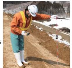
Jun Shimizume, construction department, emphasized that he can use it according to his senses of sight and hearing. "We can also stake-out by myself, without a surveyor at the instrument. We can reach the stake-out points quickly by the images of the sighting points and the guiding sound of the field controller."
